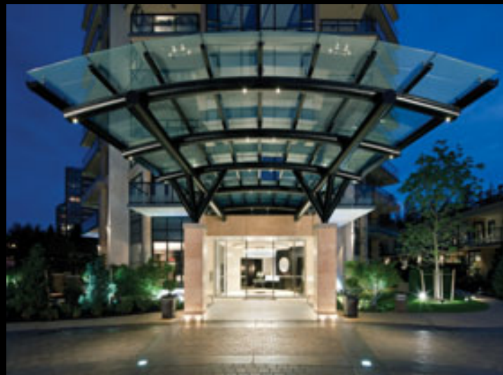
GEM OF A BUILDING: Boffo Development's Jewel tower, a finalist in several Georgie categories, overlooks Central Park in Burnaby.
